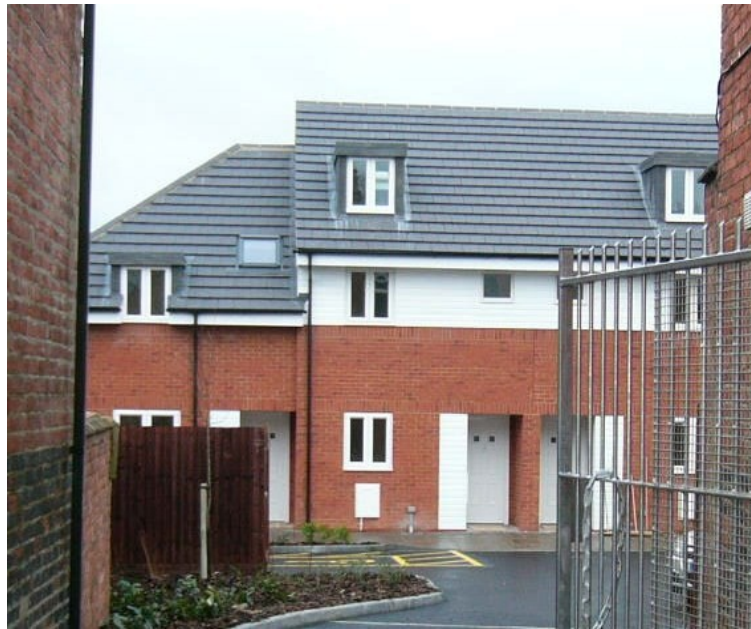
Houses at Semilong Road Northampton
