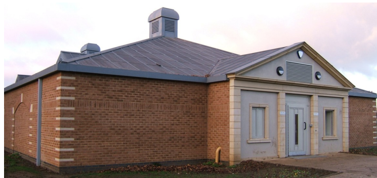
Racecourse Changing Pavilion, Northampton
