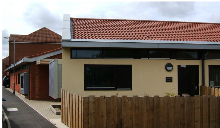
Manning Road Care Home, Moulton, Northampton
