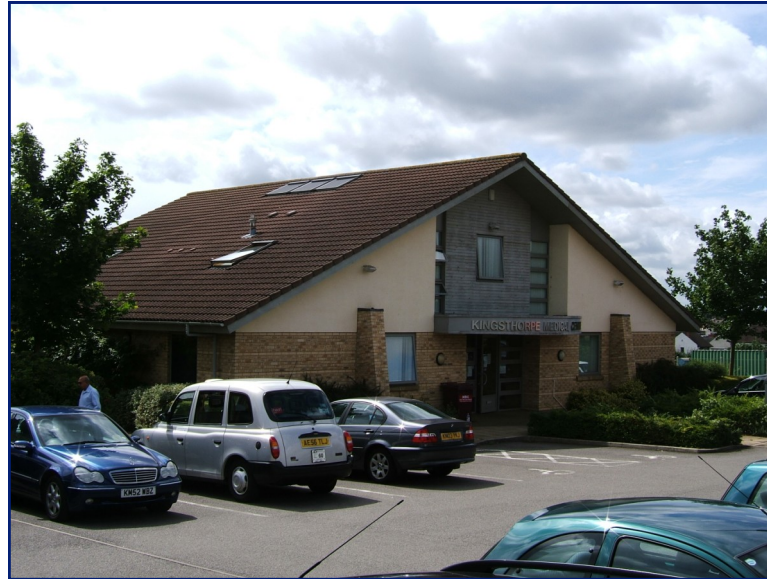
New Build Kingsthorpe Medical Centre, Northampton
