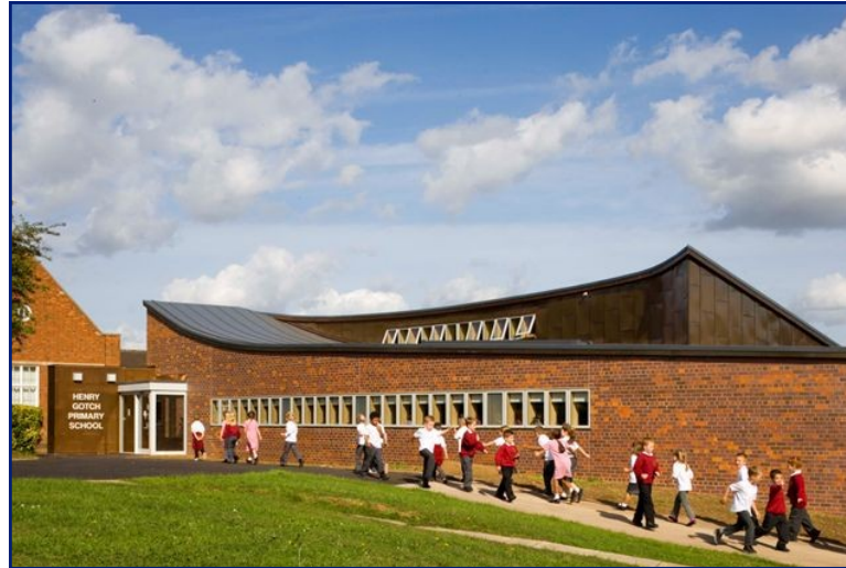
Extension to Henry Gotch Primary School, Kettering
