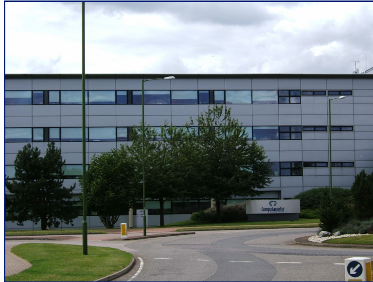
Fit out of Operations Centre & Amenity Building, Hatfield
