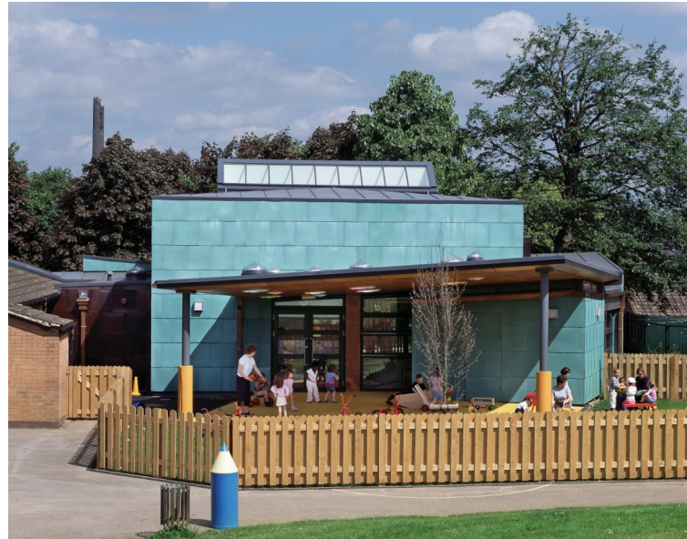
Nursery Unit at Briar Hill Lower School, Northampton
