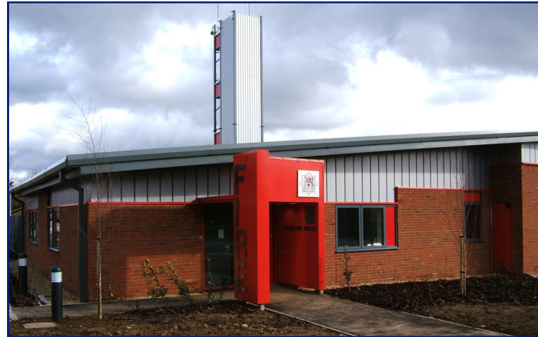
New Build—Brackley Fire Station
